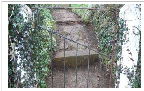
Gate repaired and path made safe
