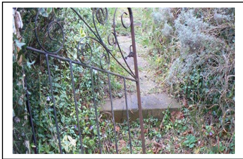
Figure 1 Gate and path unusable
